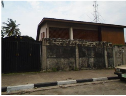
Plate 1: Photo showing a single Family Neighbourhood Source: Authors Field Work
