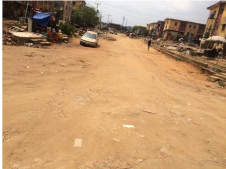
Plate 1 & 2: Isolo; The neighborhood conditions here are typical of the other case studies; collapsed roads and drains.
