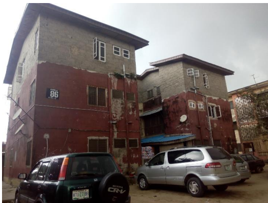
Plate 6: Amuwo Odofin- modification and addition to existing structures
