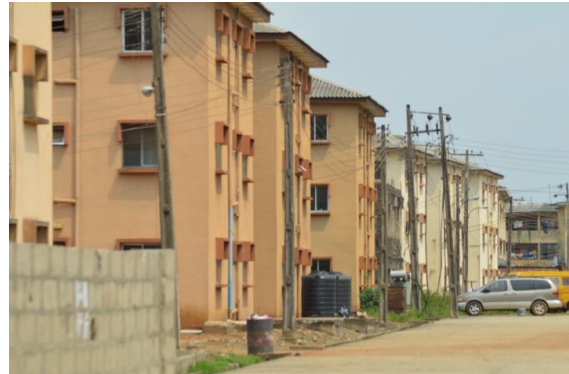
Plate 8a: Iba residential scheme. Newly built additions to residential units with improved sun-shading devices, no street sidewalks and drains.
