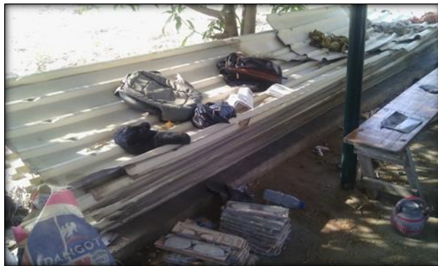
Plate 3: Roofing sheets carefully salvaged.
