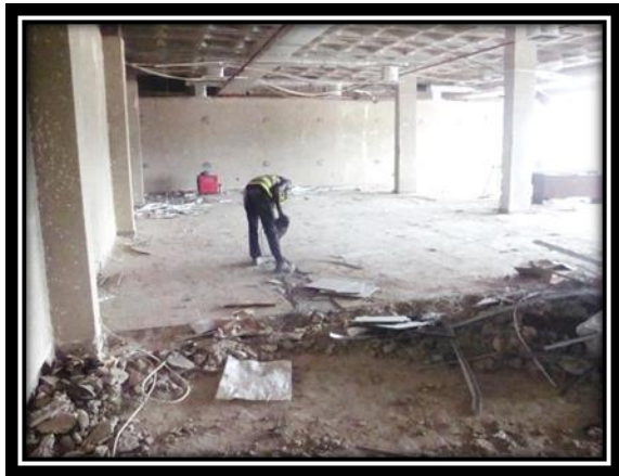
Plate 1: Removal of Floor Finish using powered tools
