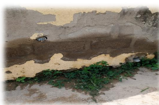
Figure 2: Blistering and flaking of mortar
