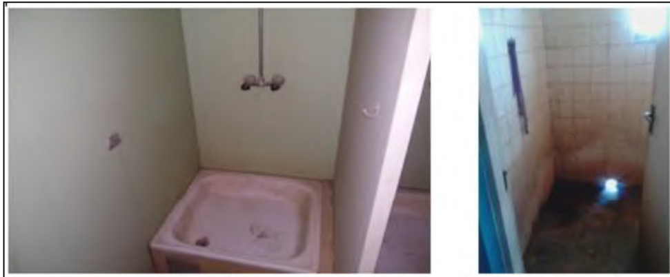
Figure 4: Example of toilet sizes provided in General hospital in Niger State
