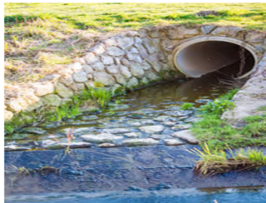
Fig. 2: Effluent drain of pond
